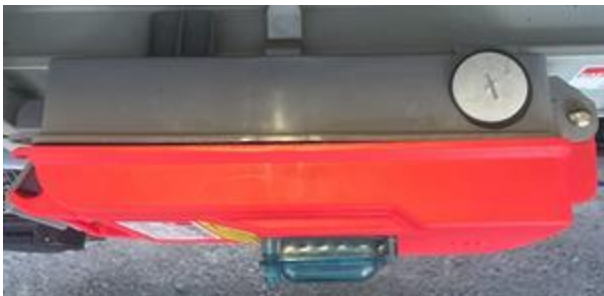
Figure 26. Tap-off Box fitted to Busbar (Top)
