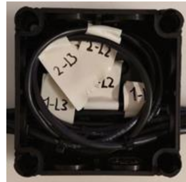
Figure 22. Looped, zip-tied and marked second set of Data cables
