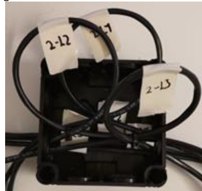
Figure 22. Looped, zip-tied and marked second set of Data cables
