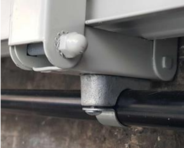
Figure 19. Conduit fixed to saddle clamp
