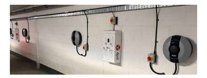
Instead, Pod Point recommended its <u>Array load balancing system</u> which works efficiently with the existing power supply to maximise the number of chargepoints that can be installed.
